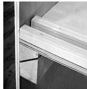
Figure 7 Horizontal panels are equipped with self-tightening French cleats on the ends opposite their mounting hinges. On this bottom panel, note the channel that houses the rear wall.
