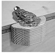
Figure 9 Draw catches secure the back panel against a strip of screen stop recessed under the top shelf.
