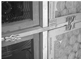
Figure 4 Turnbuttons hold the filters within screen stop ribs on the filter panel's 1x4 frame.
